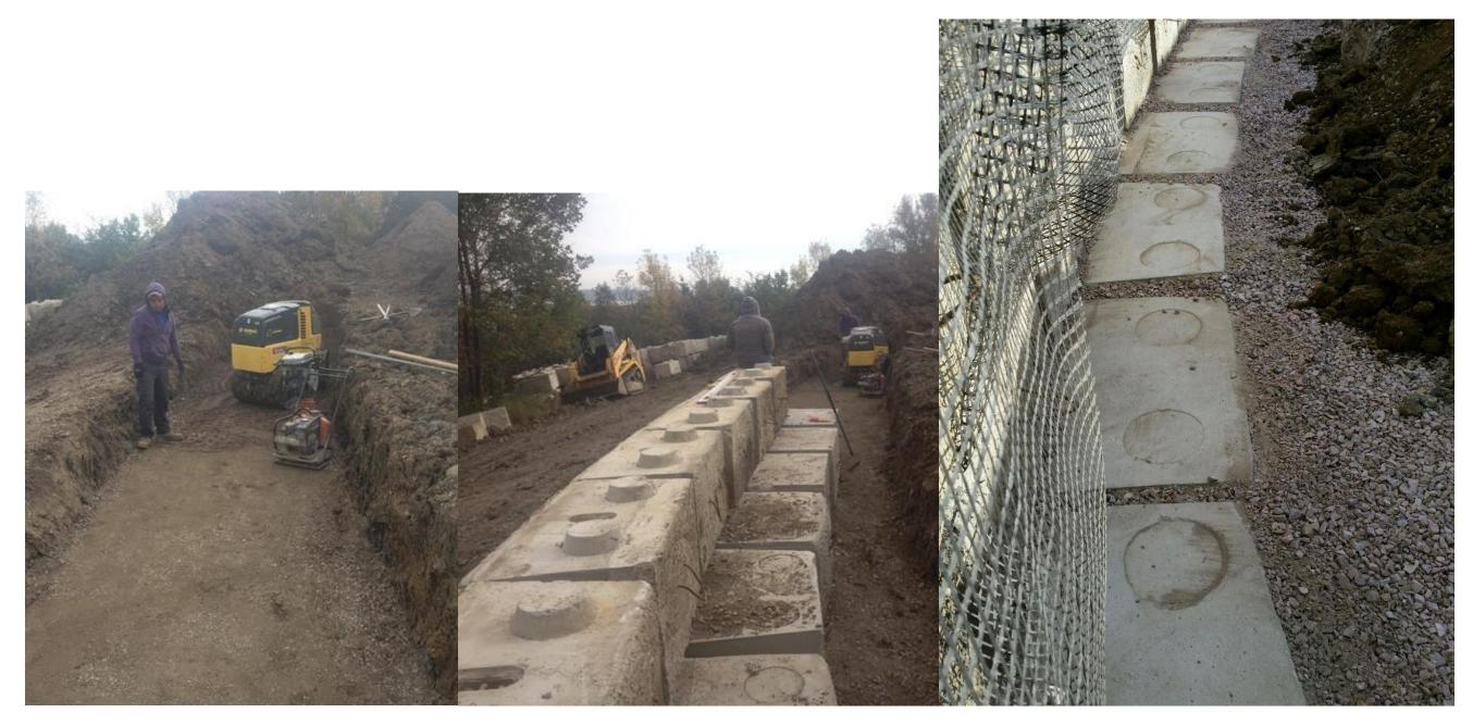
Compact your 6-8" base of gravel or crushed concrete with a packer then you can start placing your base blocks. If you are going over 8' high I would recommend using our 4400# base blocks. They will give you an excellent foundation for placing the rest of the blocks on. You may have to use more than one row of base blocks depending on your soil and height of your wall. You can also use geogrid to reinforce your wall or use a combination of both depending on your situation.
